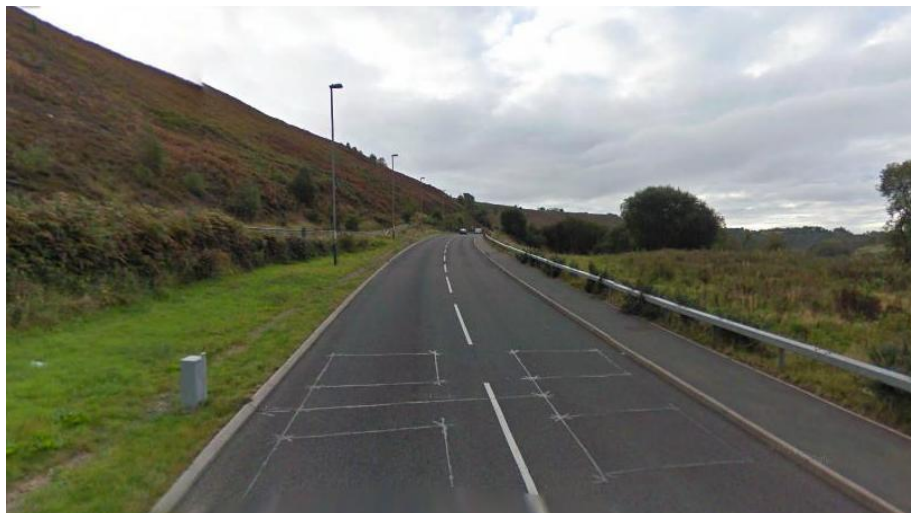
Figure F3: Southbound view between New Tredegar and Aberbargoed
