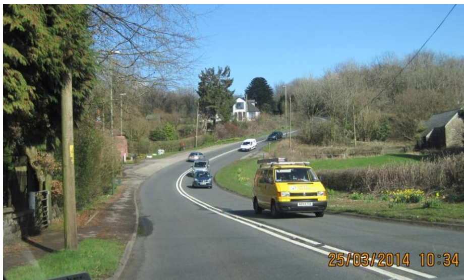
Figure C7: Northbound route near the county boundary
